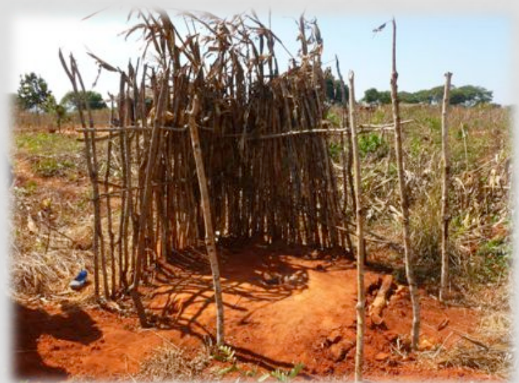
Pit Latrine without slab
