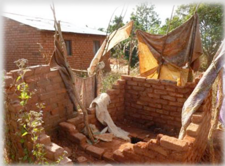
Pit Latrine with slab
